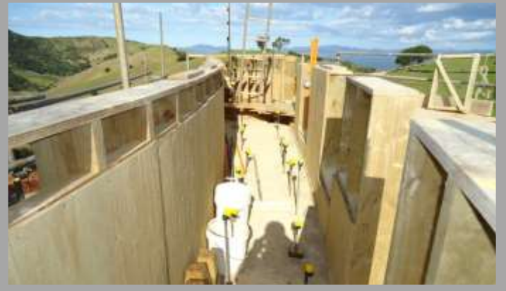
Rammed earth walls are constructed.
