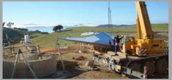
Roof is lifted into place.
